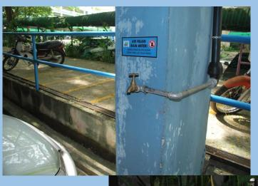
Pipes were connected to the rainwater harvesting tanks and rainwater is supplied via gravity flow.
